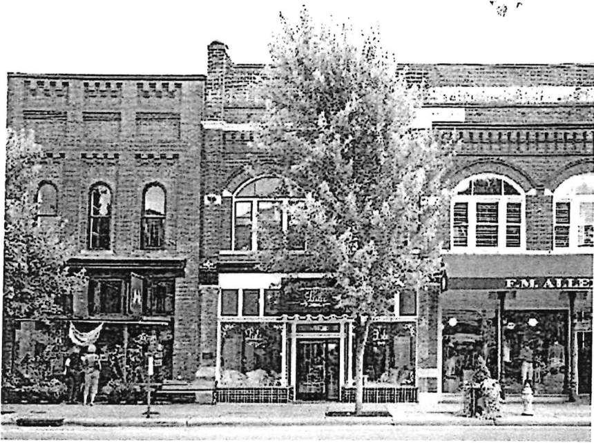
Repetition and order create a harmonious, balanced upper floor design on this building. Materials create accent and detail within a consistent palette.
