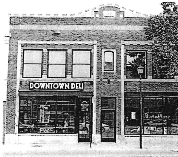
Expression lines create a vertical articulation of base, middle, and top of a facade
