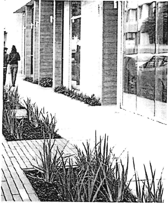
Stormwater areas and porous pavers
