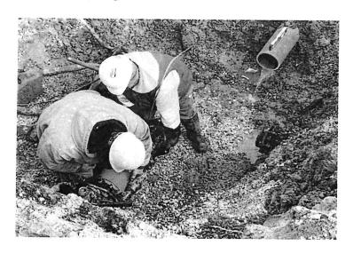
Crews filled the center of the new filter foundations and prepared the re-rod for installation of the concrete cap next week.
