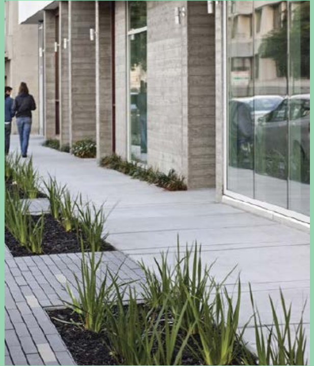
Stormwater areas and porous pavers
