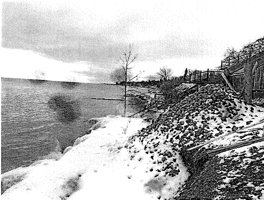
Figure 2: Photo facing south illustrating the erosion area
