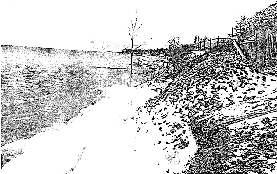
Figure 2: Photo facing south illustrating the erosion area
