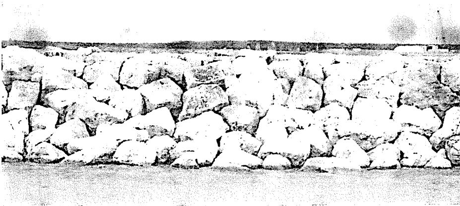
Figure 3: Shoreline revetment example
