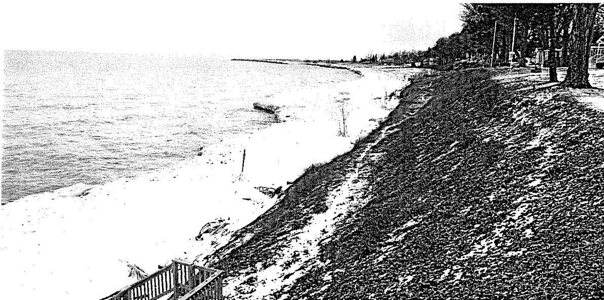
Figure 2: Photo facing southwest of steep bluff at the North
